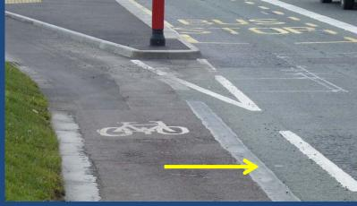
The bus stop islands have now been installed, to allow cyclists to bypass buses at normal cycling speed. The next step at this location will be to install the bus shelter and resurface the carriageway.
